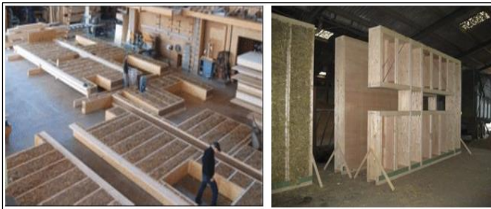
Figure 4: Straw - prefabrication with straw. Source: [6].
