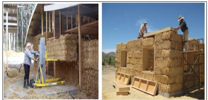
Figure 2: Straw - The post and beam system. Source: [12].
