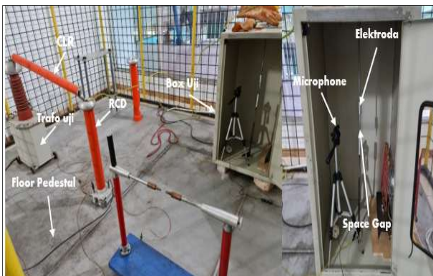
Figure 6: Research Design for Acoustic Recording of Corona Discharge in a 20 kV Cubic. Source: Authors, (2026).
