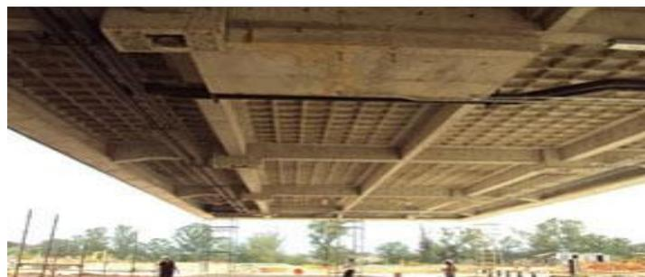
Figura 6: Lajes nervurada
