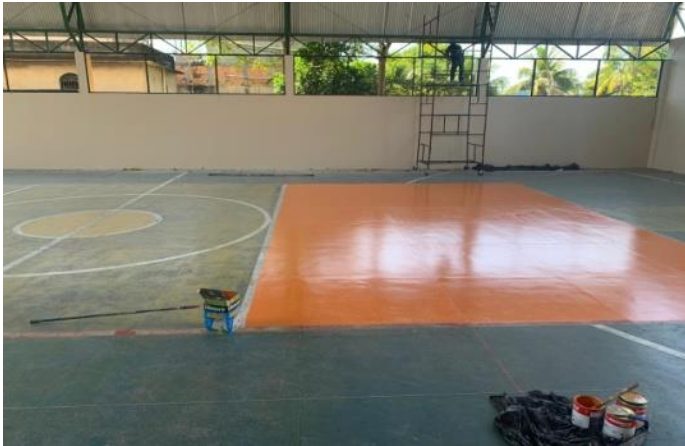
Figure 5: Worker on scaffolding in the height of 2 meters. Source: Authors, (2019).
