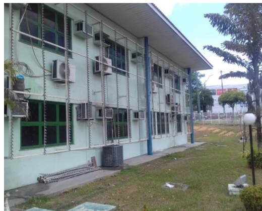
Figure 2: Facade of the Building of the UEA, Demonstration of termination of work.
