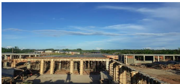
Figure 2: Slabs in Construction Process. Source: Authors, (2019).
