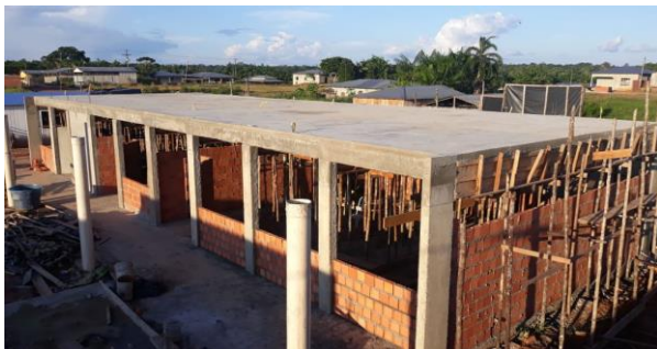
Figure 1: Construction of Slabs. Source: Authors, (2019).
