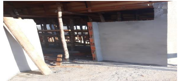
Figure 3: Slab Shoring Assembly. Source: Authors, (2019).
