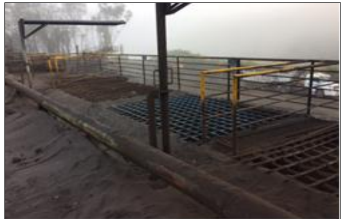
Figure 5: Silo sieves. Source: [28].
