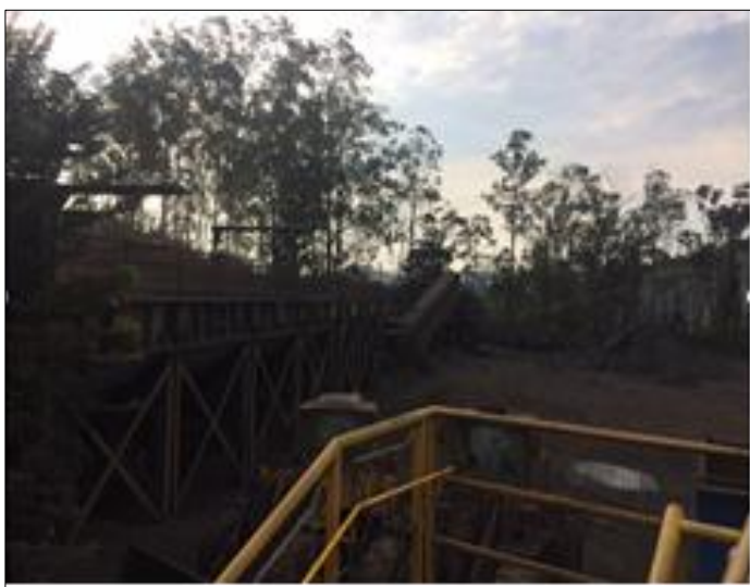
Figure 3: Partial view of the beneficiation plant (silos, conveyor belt, and homogenized material). Source: [28].
