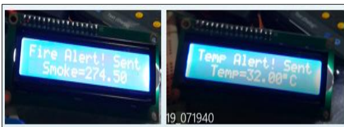
Figure 11: Alert messages on the LCD when MQ5 detected fire and DHT11 detect temperature increase. Source: Authors, (2020).
