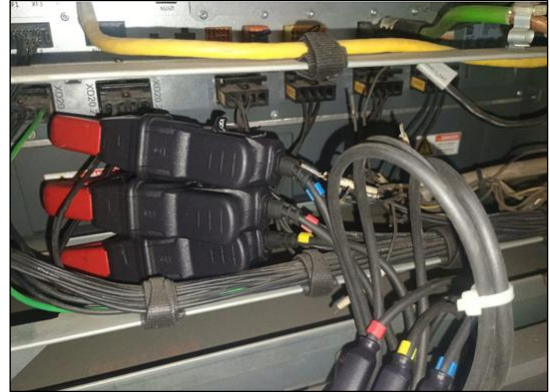
Figure 4: Installation of the CT at Axis 2 Motor of Robot in R, Y and B Phase Wires.
