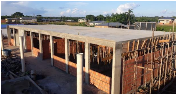
Figure 1: Construction of Slabs. Source: Authors, (2019).
