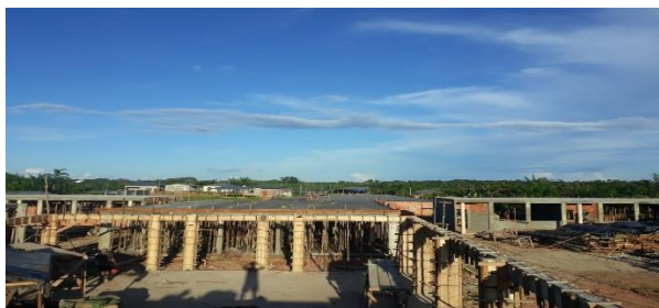
Figure 2: Slabs in Construction Process. Source: Authors, (2019).
