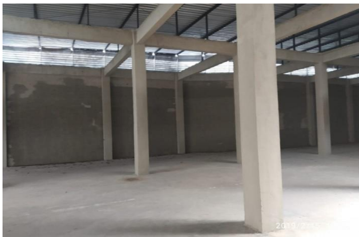
Figure 4: Company Interior. Source: Authors, (2019).
