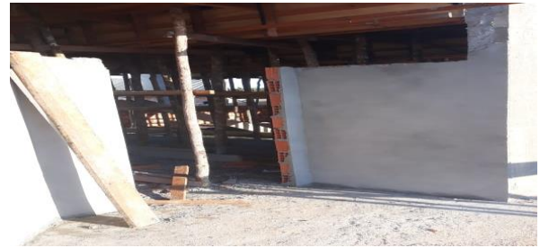
Figure 3: Slab Shoring Assembly. Source: Authors, (2019).
