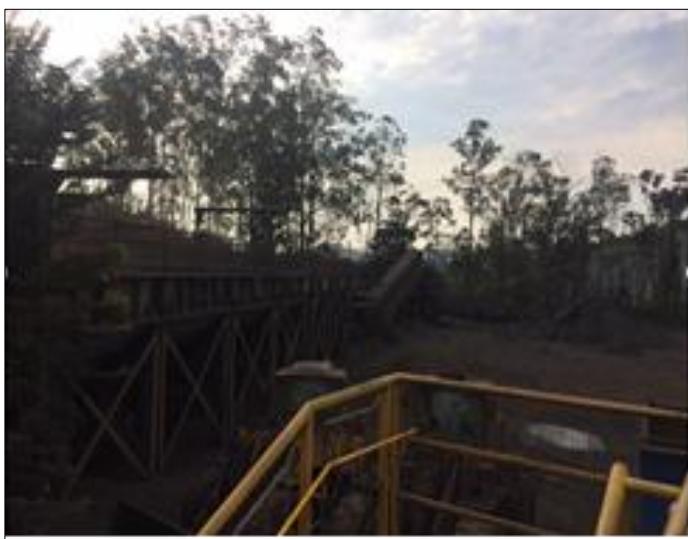
Figure 3: Partial view of the beneficiation plant (silos, conveyor belt, and homogenized material). Source: [28].
