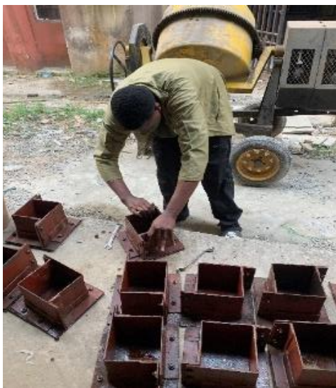
Figure 11: Cleaning of moulds to receive mixed concrete. Source: Authors, (2025).
