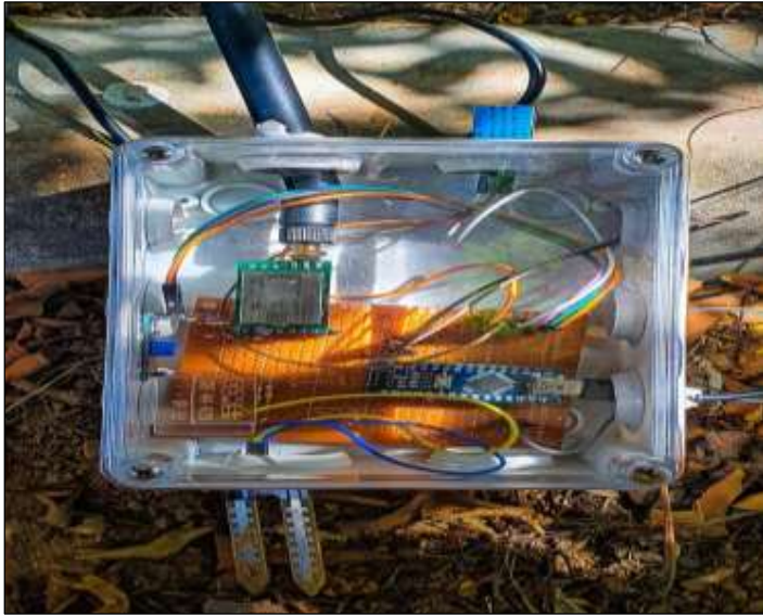
Figure 8: actual deployment of the field node. Source: Authors, (2025).
