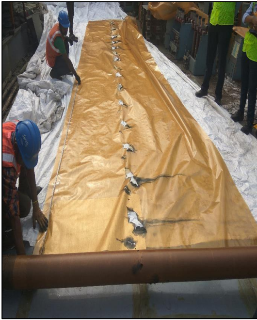
Figure 4: Radial Breakdown of bushing paper near the bushing flange. Source: Author, (2026).
