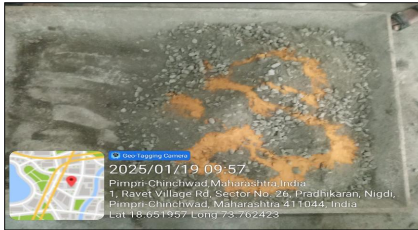
Figure 2: Addition of TGB during preparation of concrete. Source: Authors, (2026).
